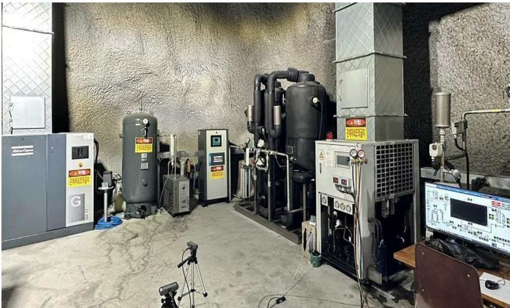
Figure 3. The layout of the custom-made Radon Reduction System. 1: Compressor, 2: Receiver tank, 3: Absorption dryer, 4: Air chiller, 5: Heater and HEPA filter units, 6: Active charcoal tanks, and 7: Control panel.
