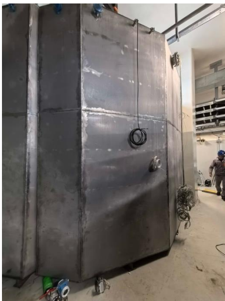
Placement of water tank Dry run ongoing
