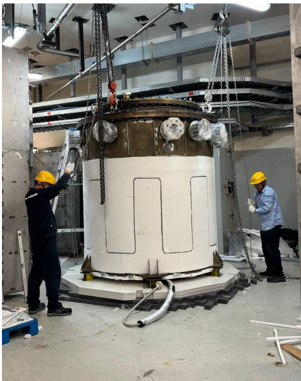
Placement of stainless steel tank
