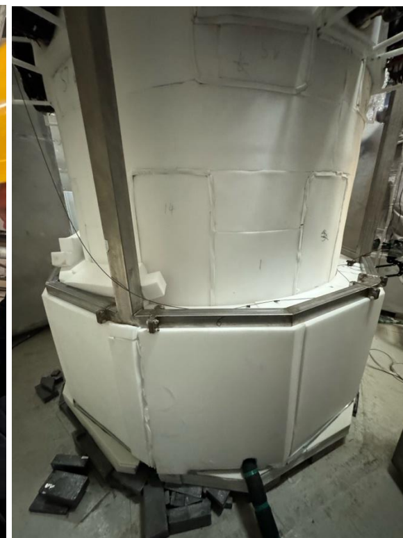
Assembling of thermal insulation (Melamine foam)
