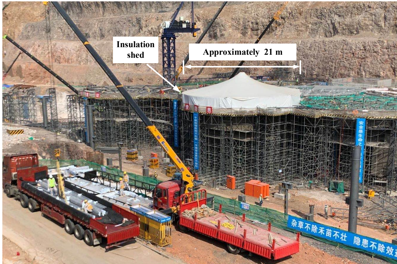
Construction site of Nanjing Future Garden
